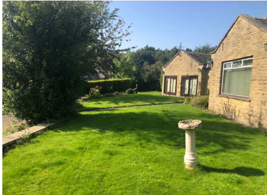
Front southern elevation
