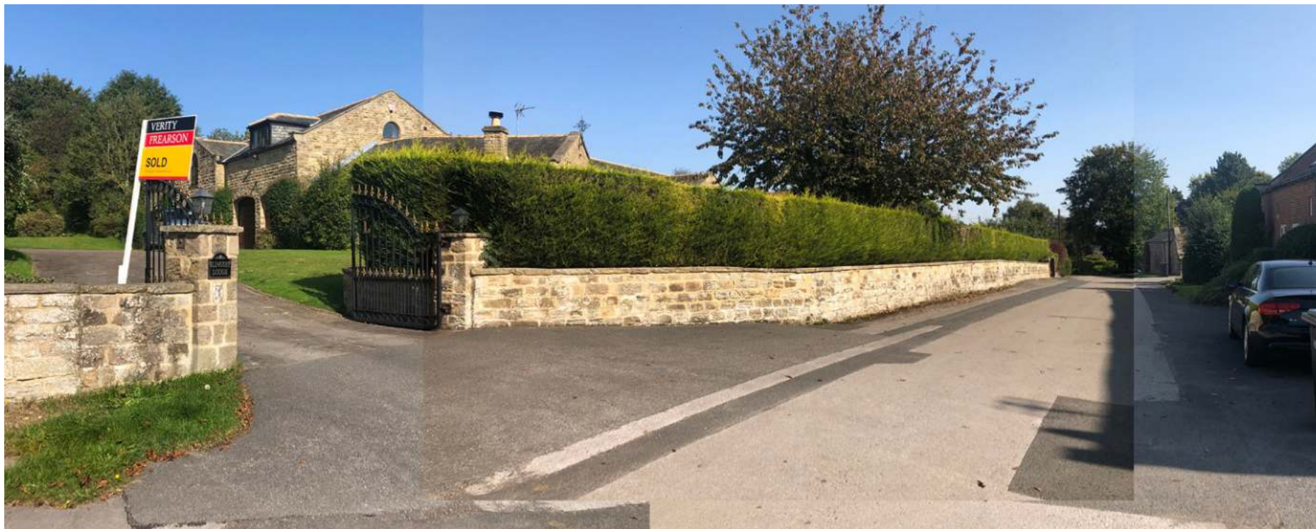
View of entrance driveway and stone wall mentioned in the conservation area appraisal
