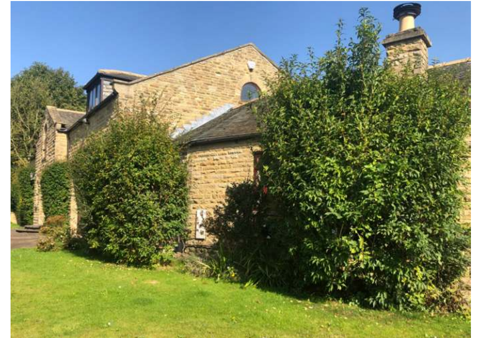
Oblique view along west elevation
