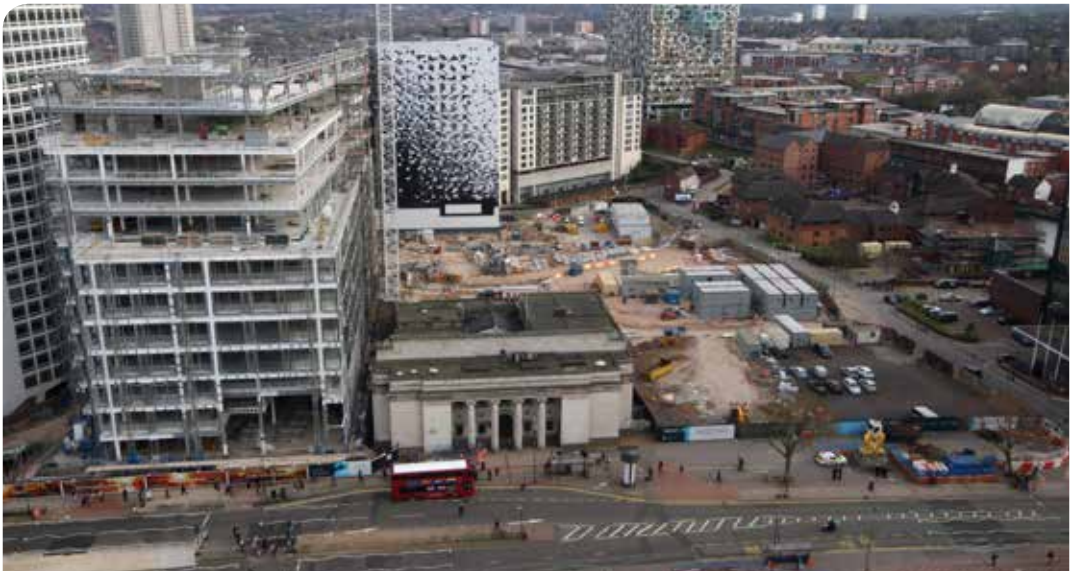
VIEW OF WORKS FROM THE LIBRARY OF BIRMINGHAM
