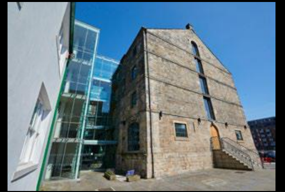
CARVERS WAREHOUSE, MANCHESTER
