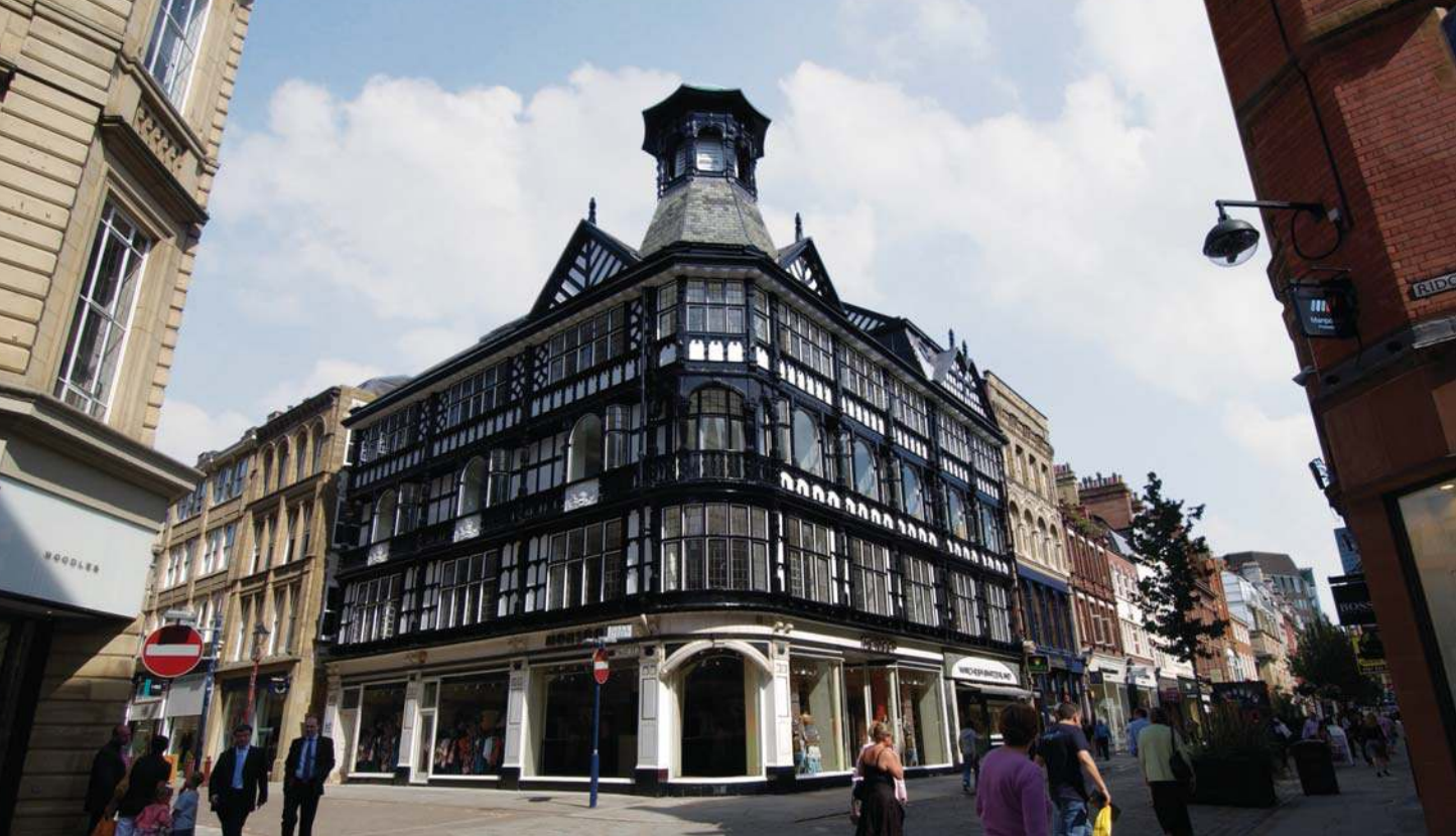
A prominent location at the corner of King Street & Police Street
