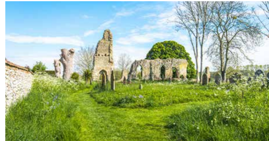
Church ruins on Raynham Estate
