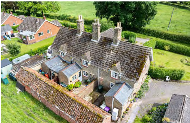
Rear View of the Cottages
