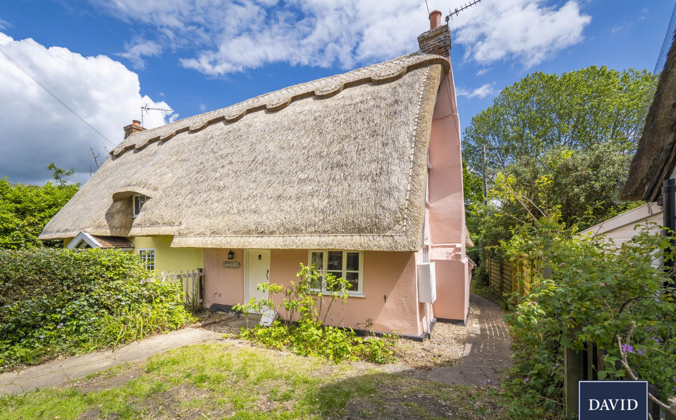
Windfall Cottage, The Row, Hartest, Suffolk
