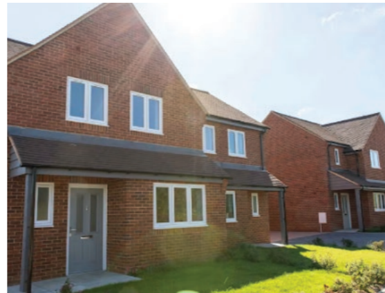
Beech Farm, Postcombe Completed November 2020
