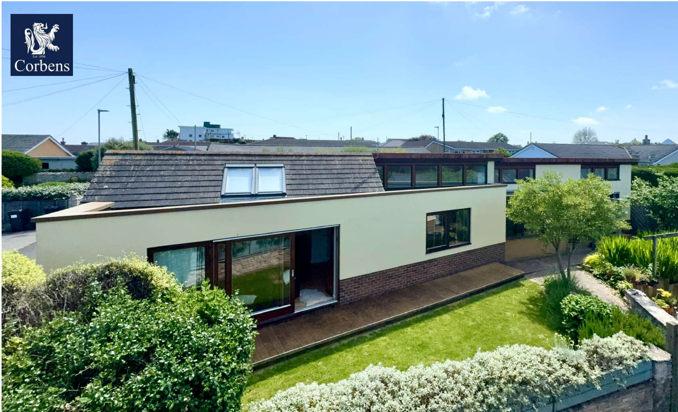
THE WEDGE, 39 BALLARD ESTATE, SWANAGE £995,000
