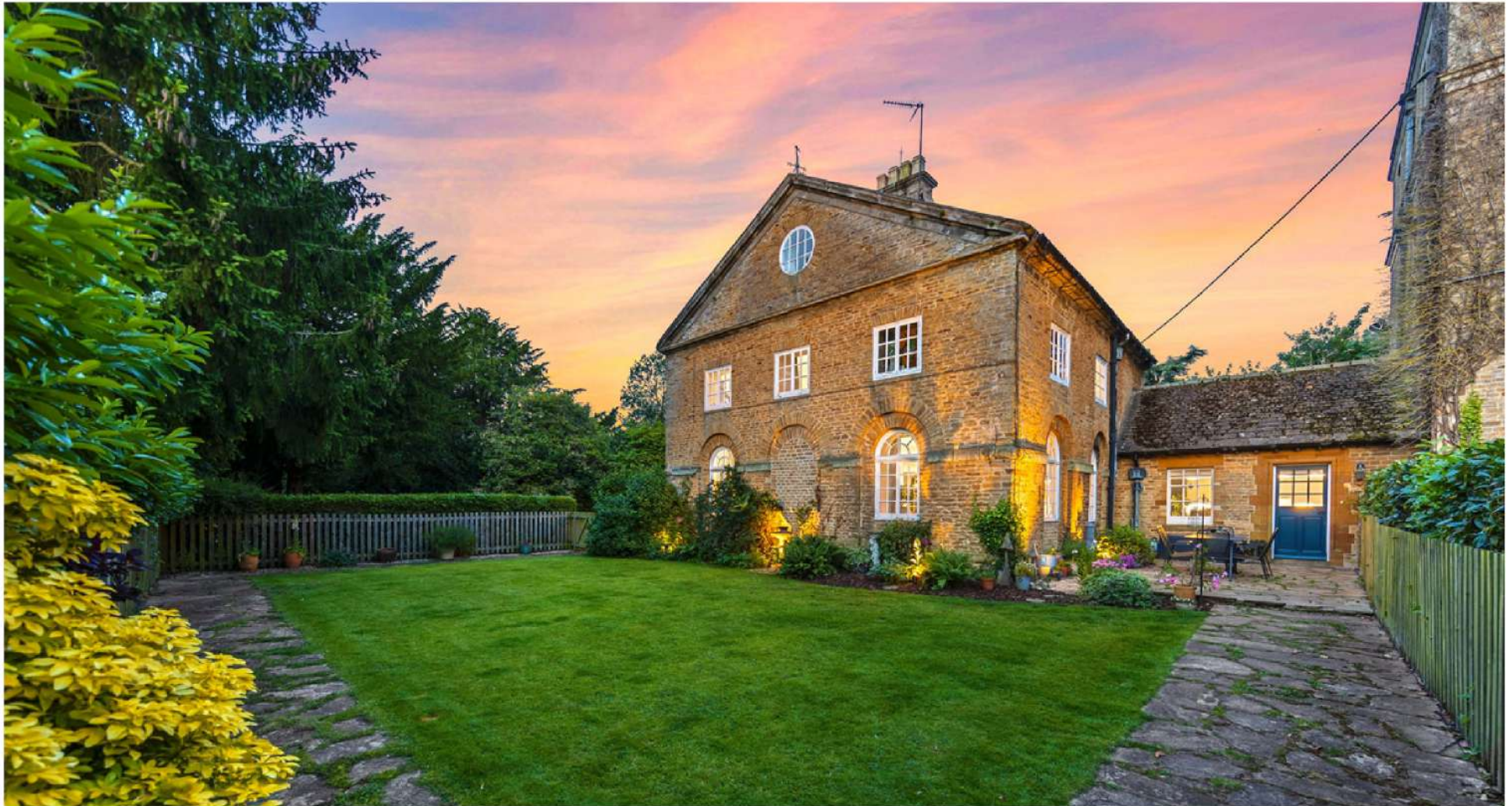
The Dower House, Pitsford Hall, Moulton Road, Pitsford, Northampton, Northamptonshire, NN6 9AU
