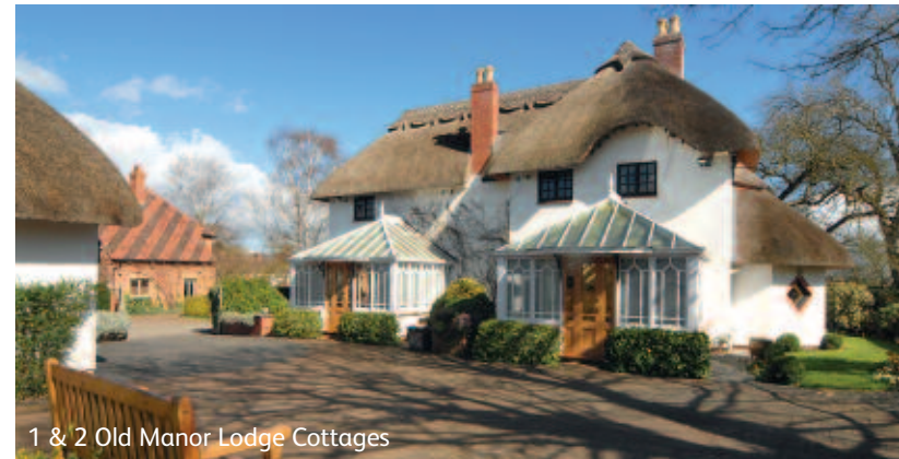
2 Old Manor Lodge Cottages
