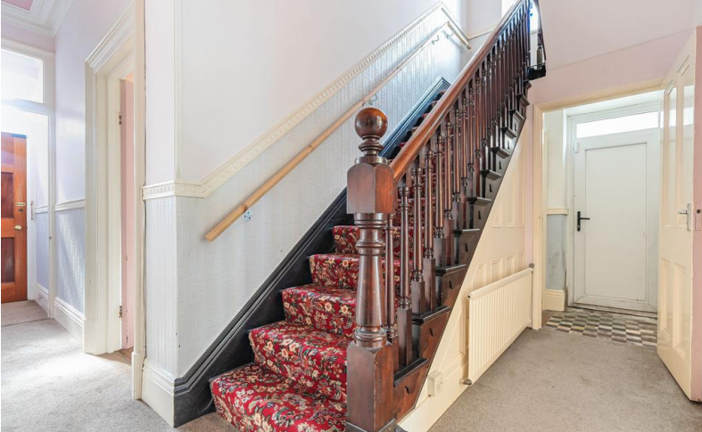
Hallway and Stairs
