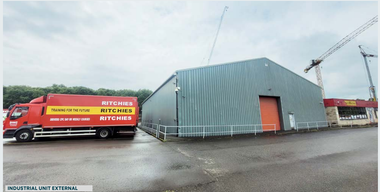
INDUSTRIAL UNIT EXTERNAL
