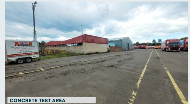
CONCRETE TEST AREA
