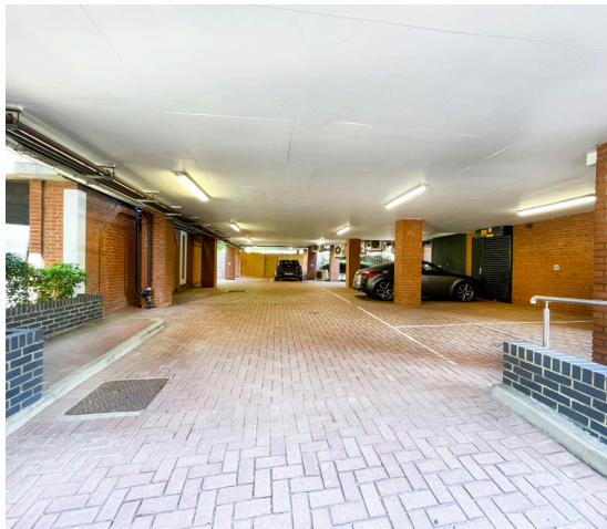
Undercroft car park
