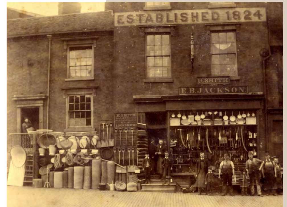
A Victorian photograph of the 'newly established' Harry Smith ironmongery.
