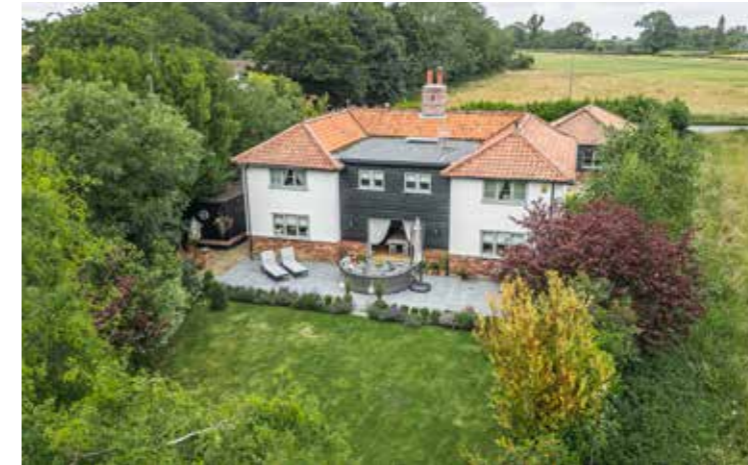
Rear of Green Cottage.
