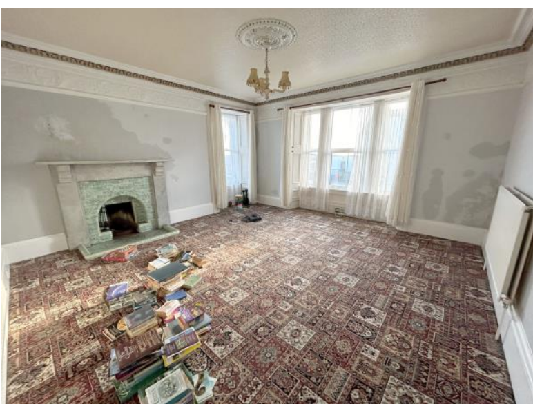
First Floor Lounge
