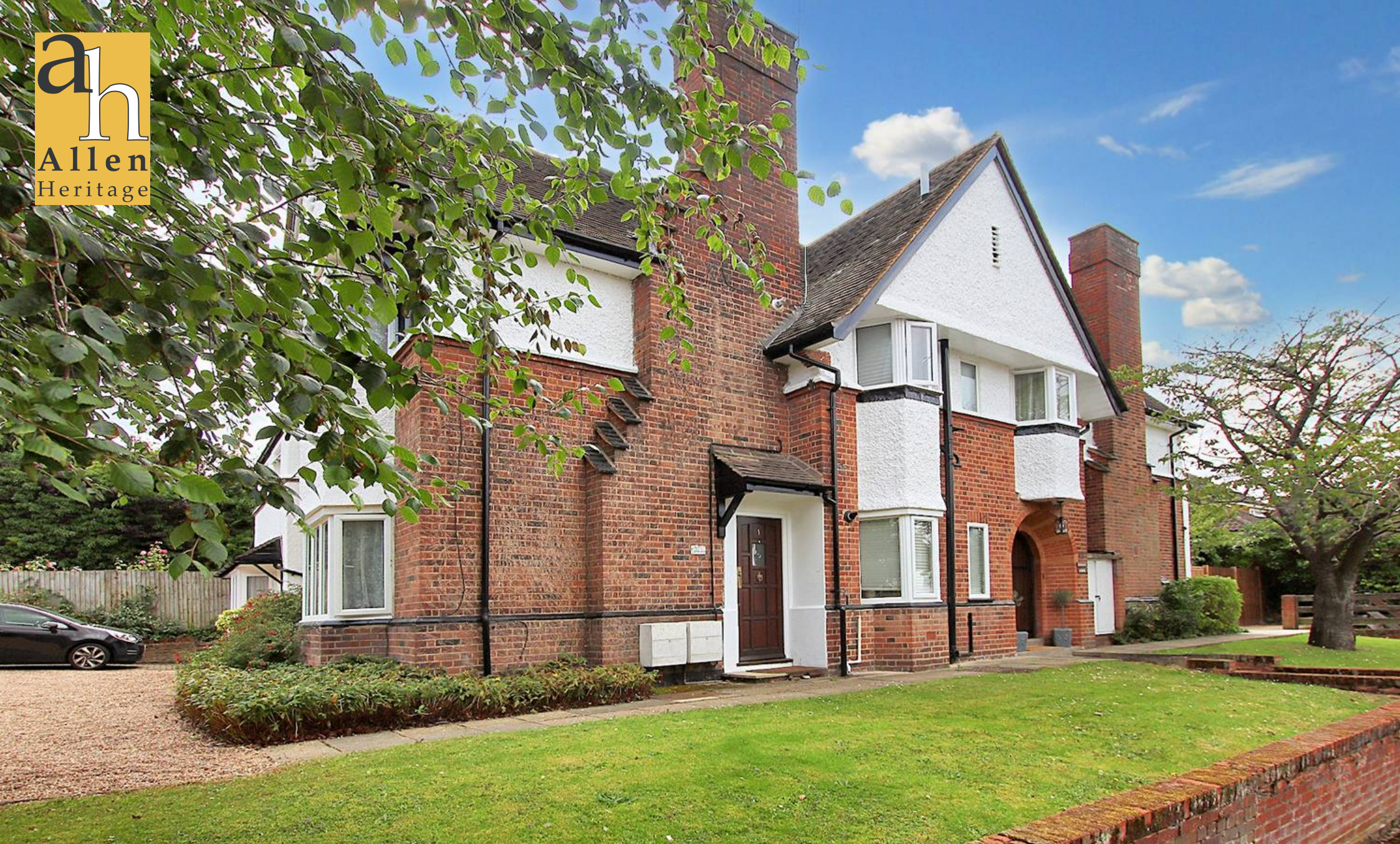
Flat 2, Durham Lodge, 12 Durham Avenue, Bromley
