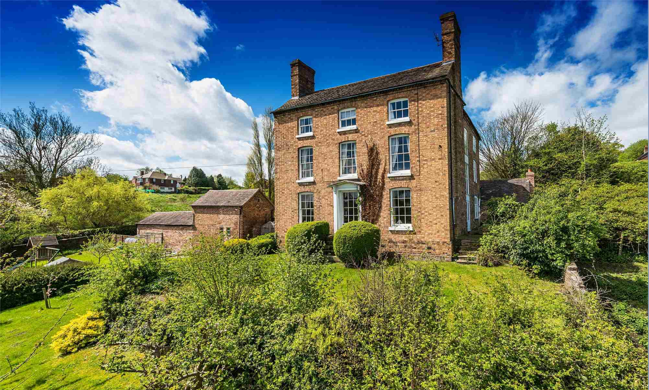
Hilltop House, Bridge Road, Benthall, Broseley
