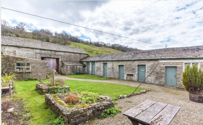
Outbuildings and Barn
