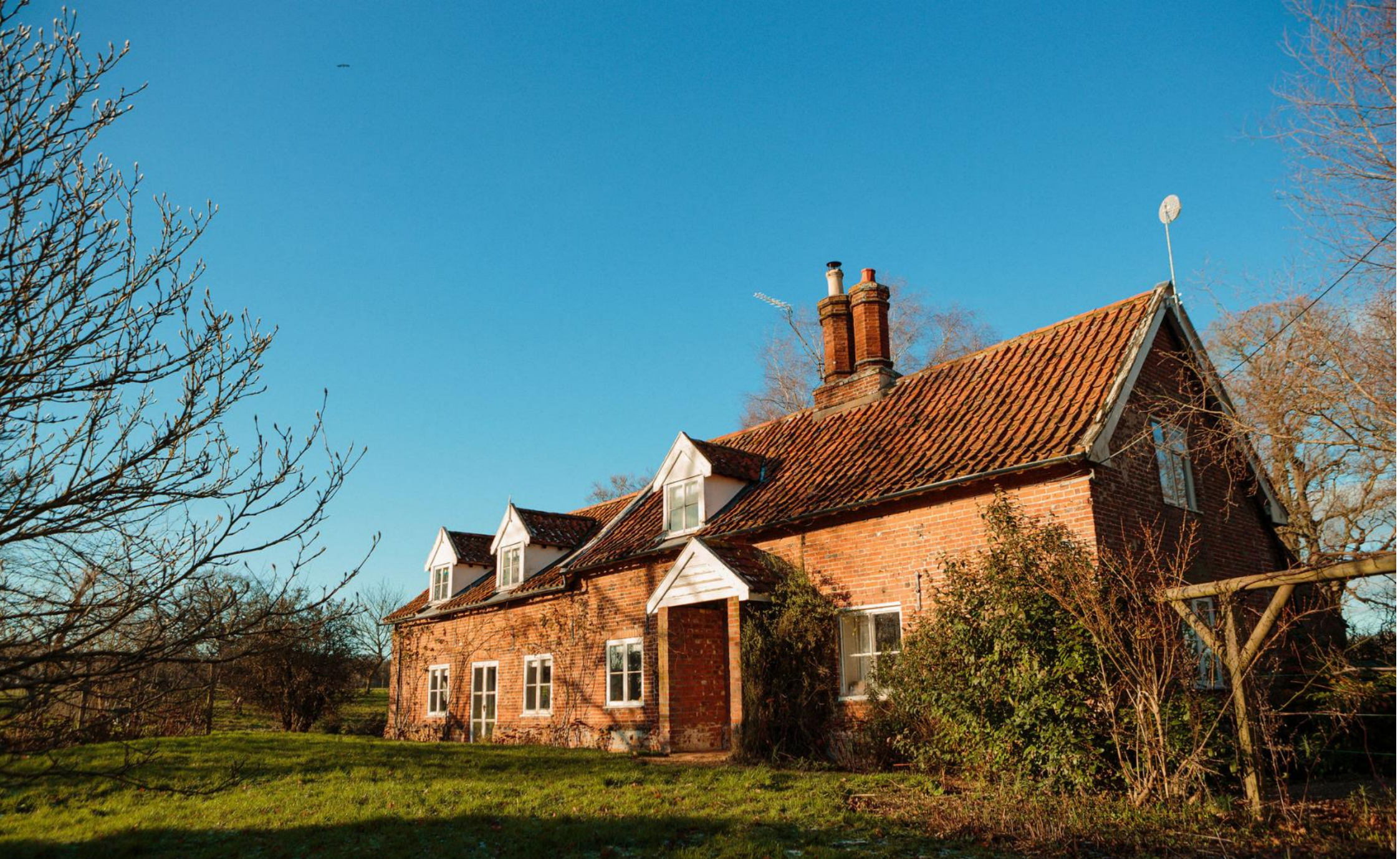
Keepers Cottage, Wolterton Hall
