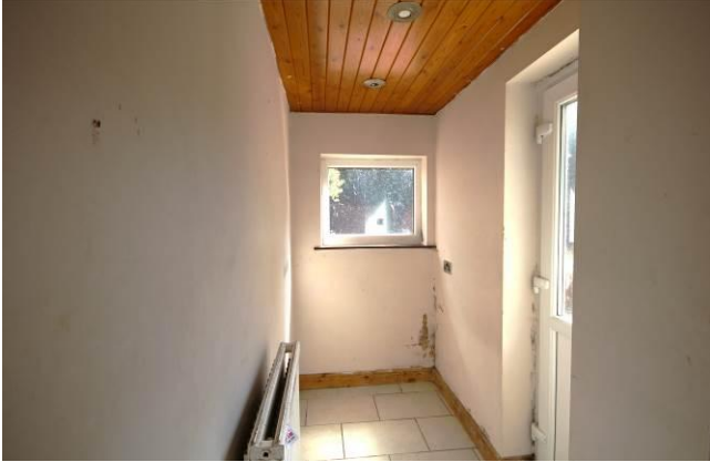
STAIRS AND LANDING: Inset spot lights. Coved and Textured Ceiling.
