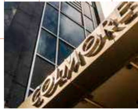
COLMORE GATE AT COLMORE ROW
