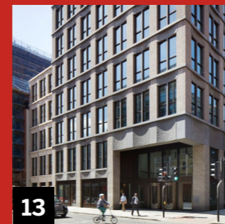
13 FEATHERSTONE BUILDING, EC1 Developer: Derwent London Size: 124,000 sq ft Status: Completed Q2 2022 95% let
