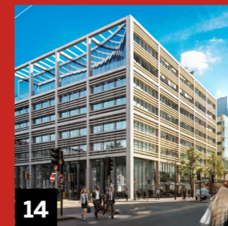
14 50 FINSBURY SQUARE, EC2 Developer: GPE Size: 117,300 sq ft offices Status: Completed 2021 Prelet to Inmarsat
