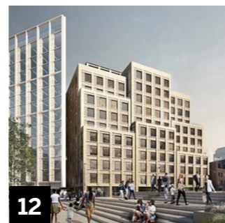
12 BLOSSOM STREET ESTATE, E1 Developer: British Land Size: 347,000 sq ft office, 40 luxury apartments & 2 public squares Status: Completed 2024
