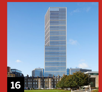
16 HYLO 103 - 105 BUNHILL ROW, EC1 Developer: CIT Size: 261,143 sq ft offices Status: Completed Q4 2021 90% let
