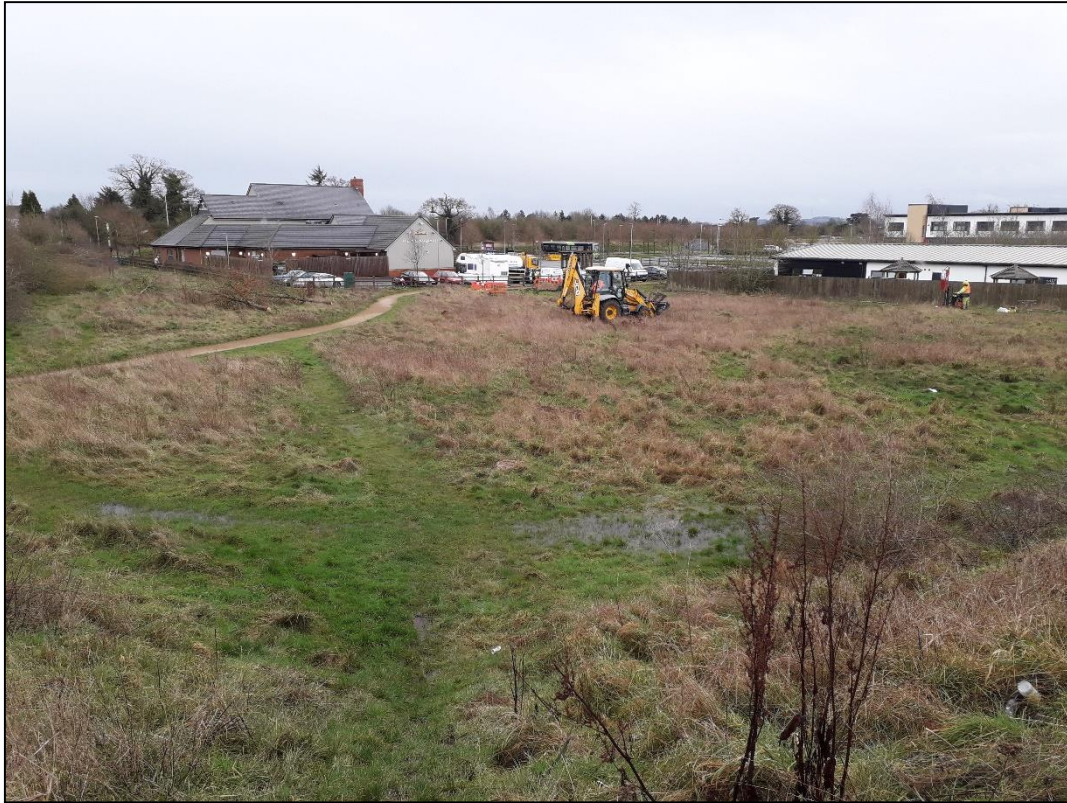
View across site from top of western bank showing public house (left) and waterlogged ground (centre)
