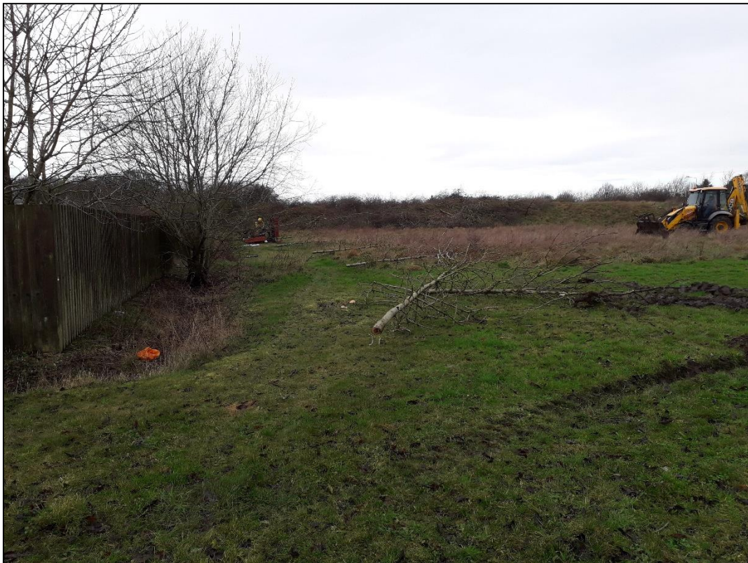
View along southern site boundary with nursery school (view to west)
