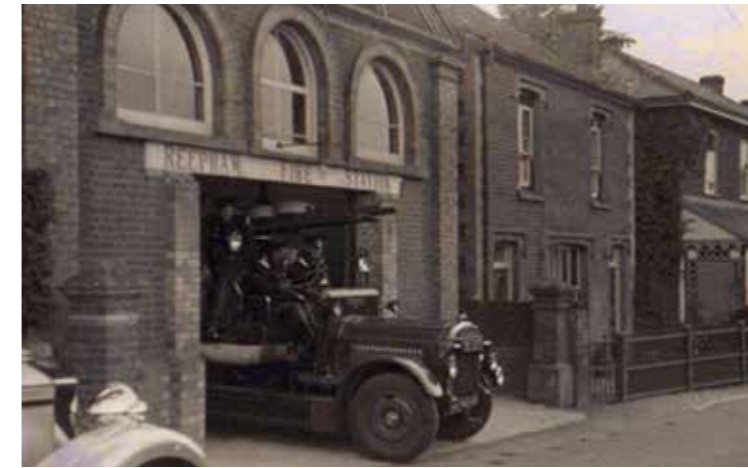
Reepham Fire Station, 1936.
