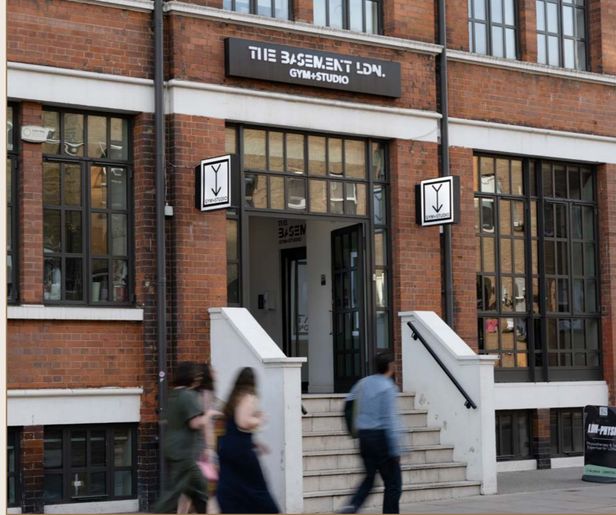
The Basement LDN Gym + Studio
