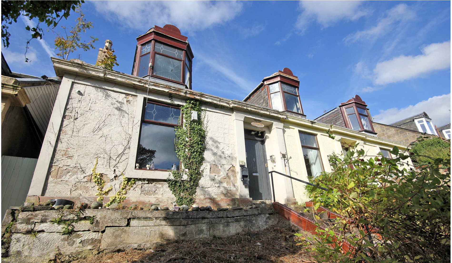
12 Dean Terrace, Kilmarnock KA3 1RJ Offers Over £75,000
