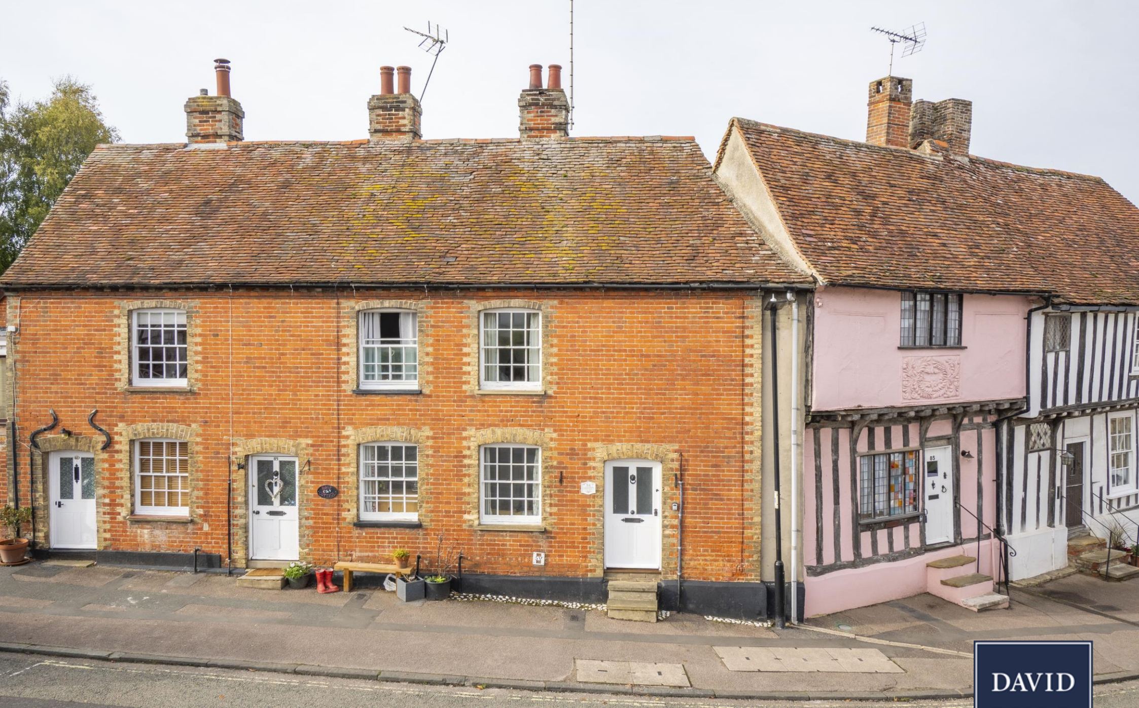
Lavender Cottage, 84 Church Street, Lavenham, Suffolk
