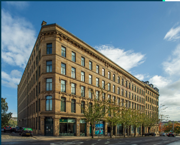
Broadgate House, Broad Street, Bradford, BD1
