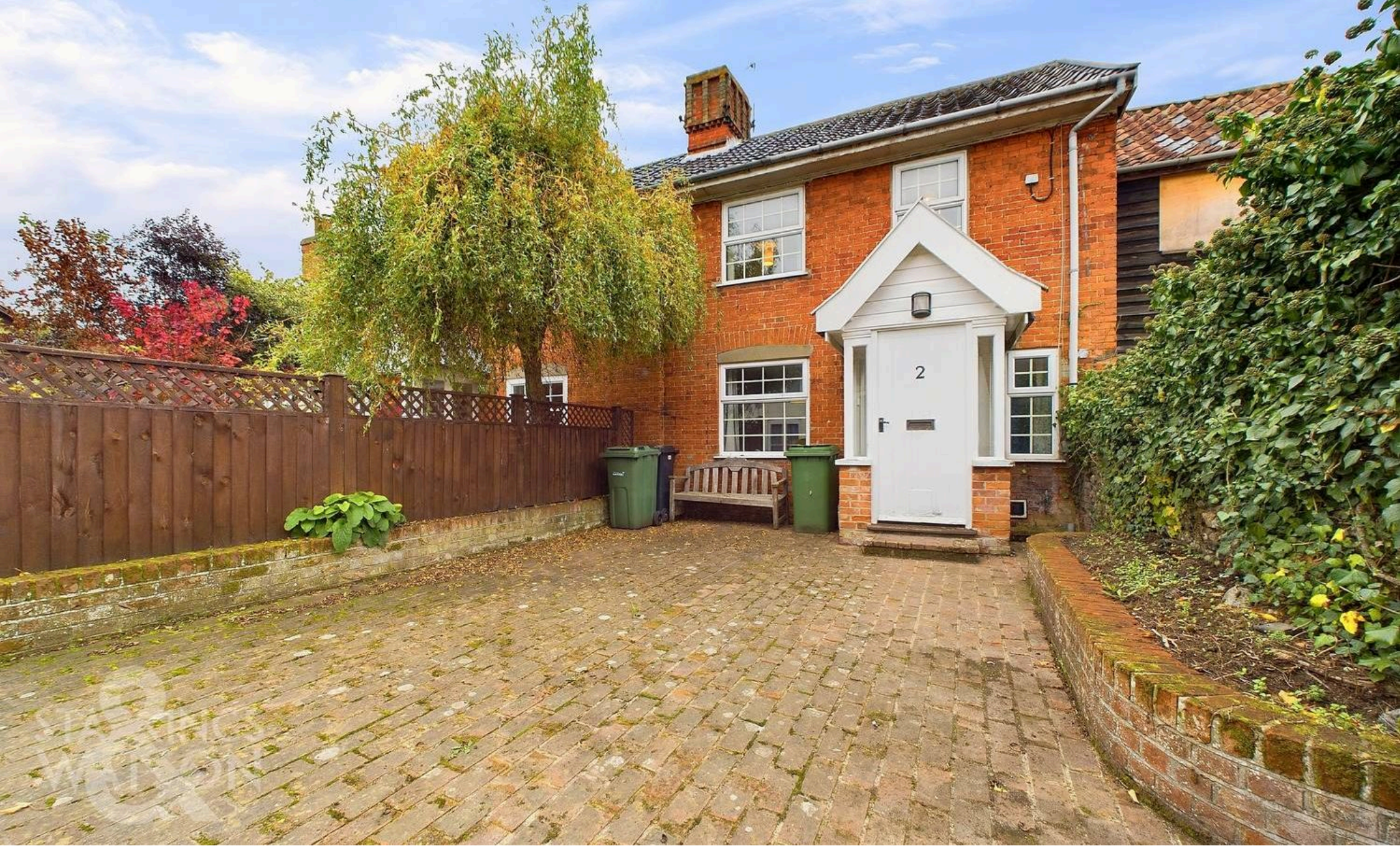
Old Chapel Yard, Harleston - IP20 9AJ
