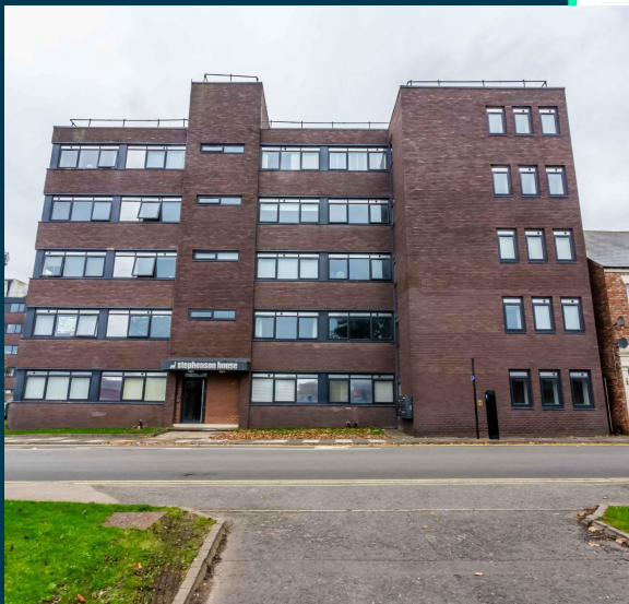
Stephenson House, Stephenson Street, North Shields, NE30 1QA
