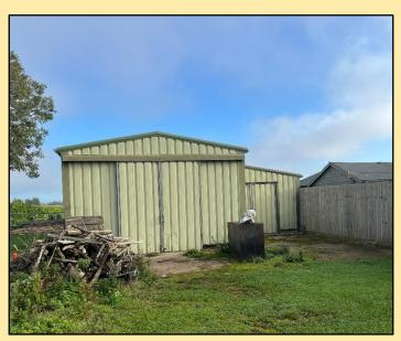
The area comprises of two parts being the main building and a lean-to. The main part comprises of a steel portal framed structure with plastic profile coated metal sheeting to the sides and an internal block wall to approximately 1.5 meters high with a pitched big six sheeted roof over. The lean to is situated to the East of the main building and comprises of similar construction to the main building. The total site area extends to 0.047 Hectares (0.116 Acres) or thereabouts.
