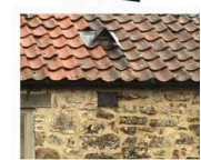
lead vent tile (in clay Pantile)
