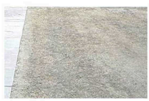
bound gravel (perimeter paths)
