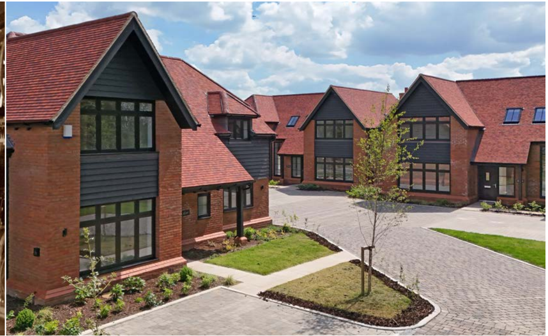
The Green at Owlswick in Buckinghamshire - an exclusive luxury development completed in 2024
