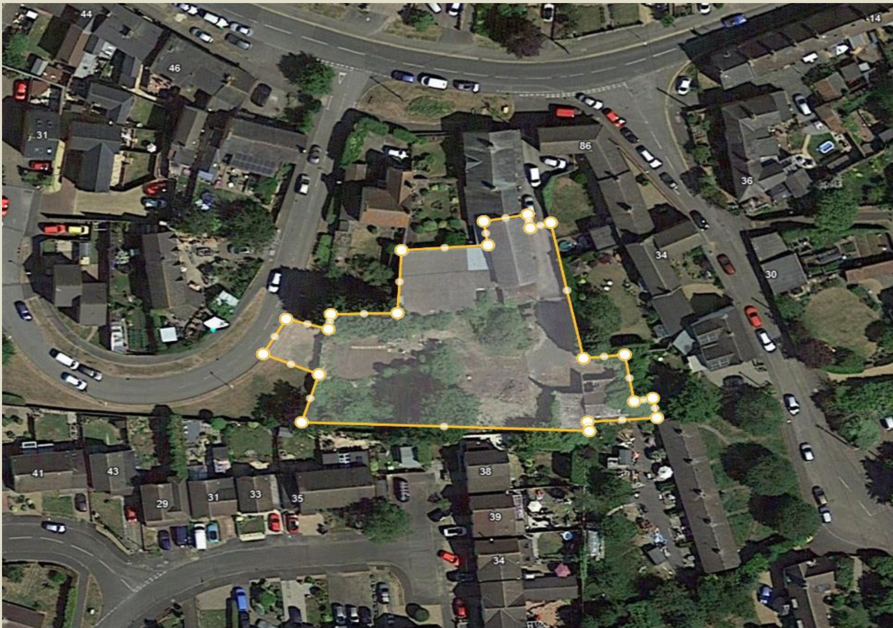
Site Location Google Map – the site is cleared from trees and vegetation
