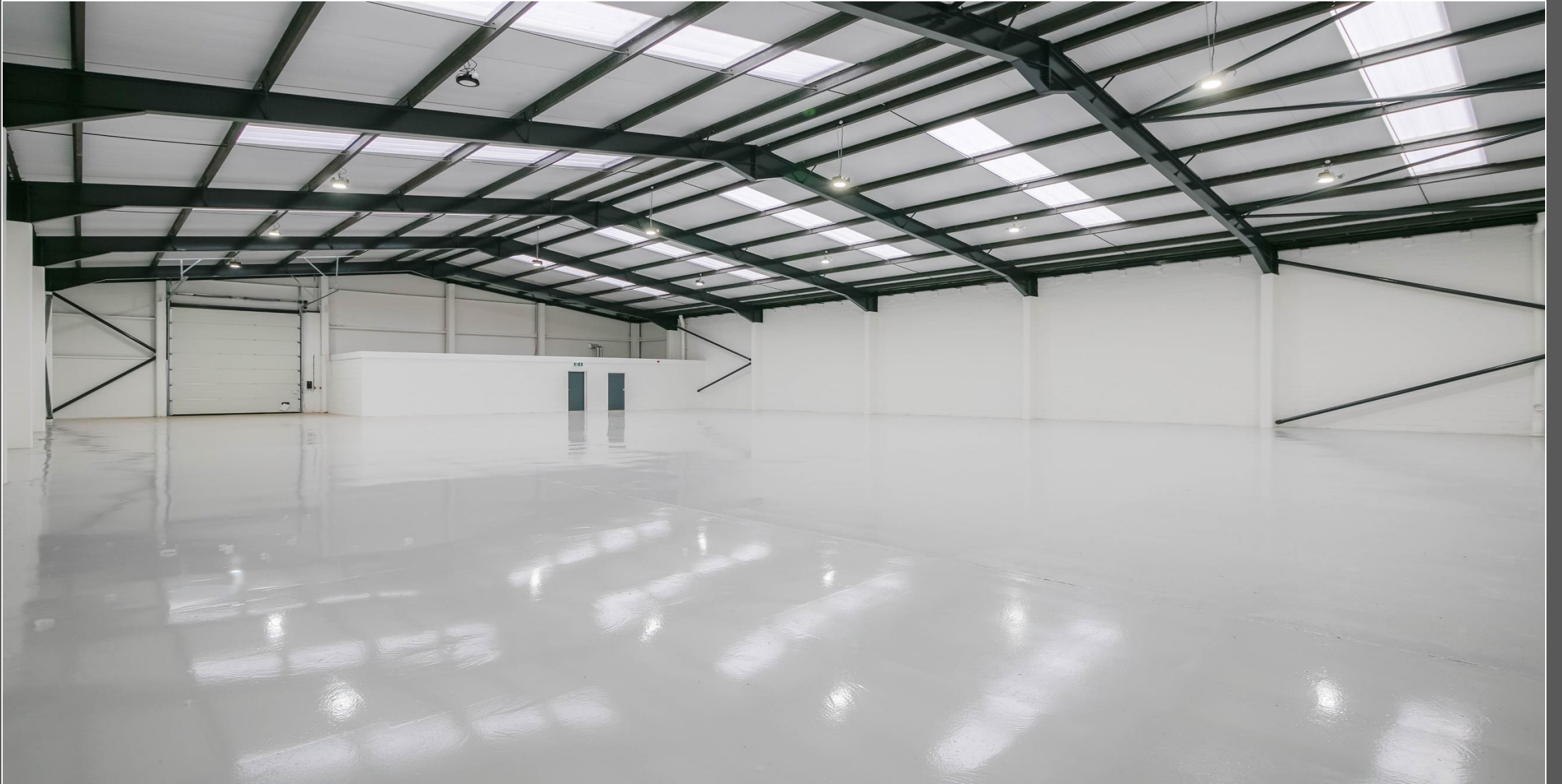
Ground Floor Clear Span Warehouse/Industrial Area (Image taken in 2022)
