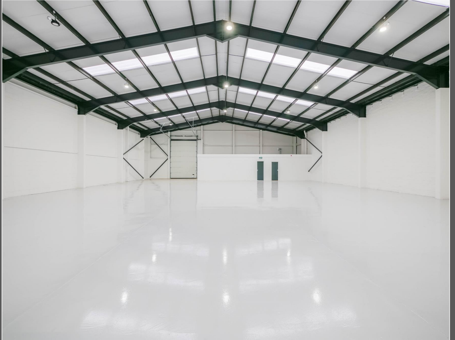
Ground Floor Clear Span Warehouse/Industrial Area (Images taken in 2022)
