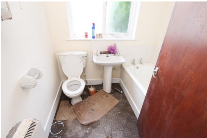
Adjoining cottage bathroom
