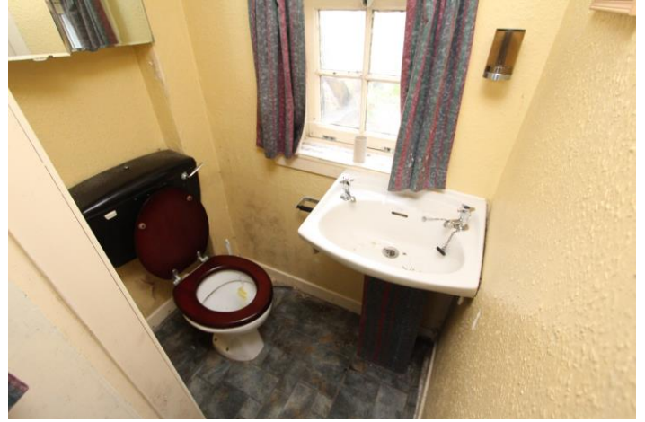
Basement flat WC
