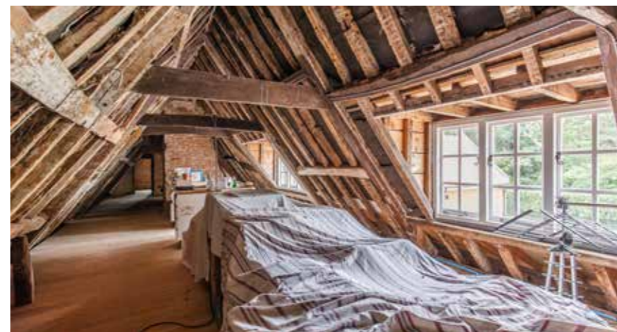
The attic space at Humbletoft.
