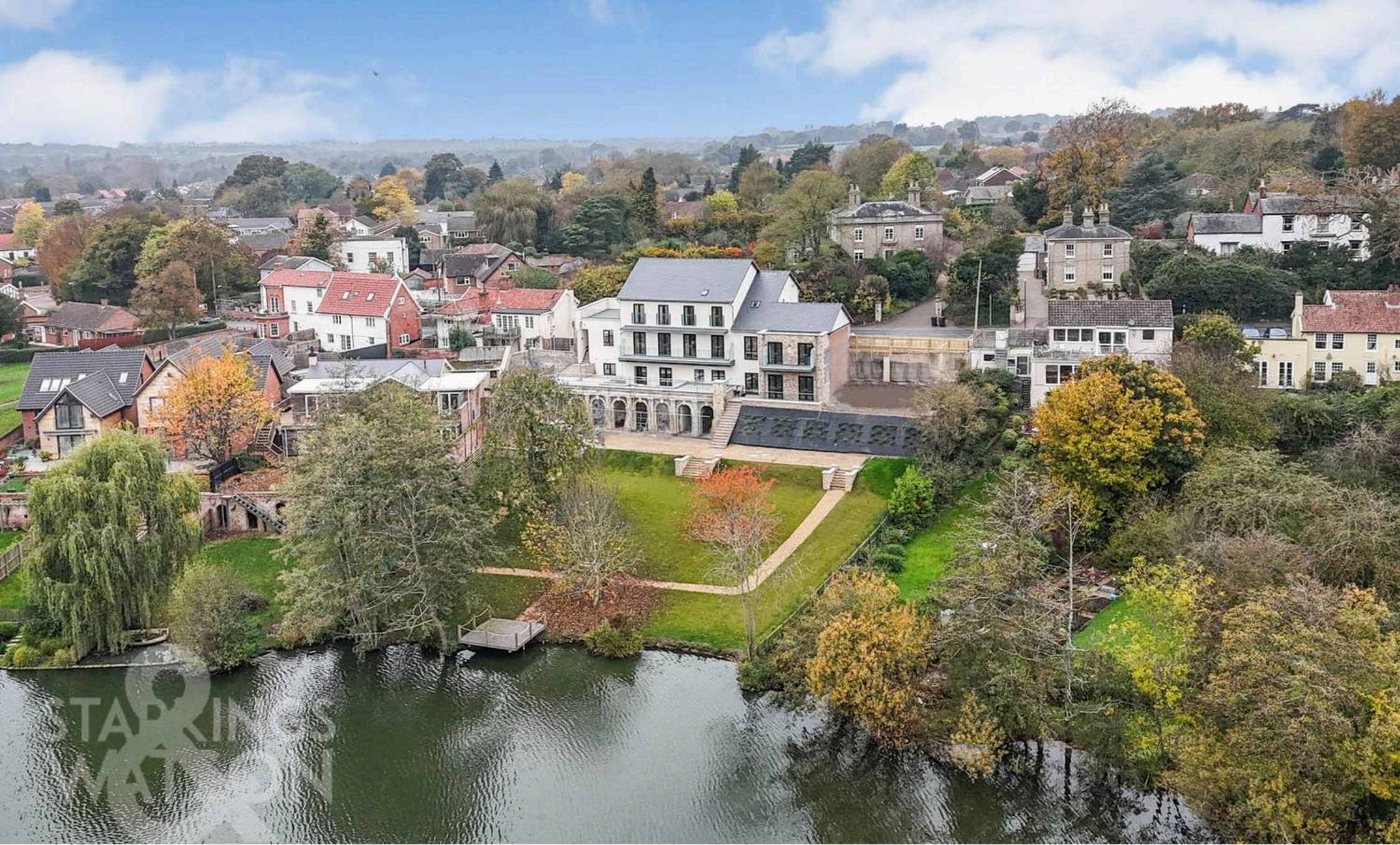
Grasmere Apts, Denmark Street, Diss - IP22 4LE
