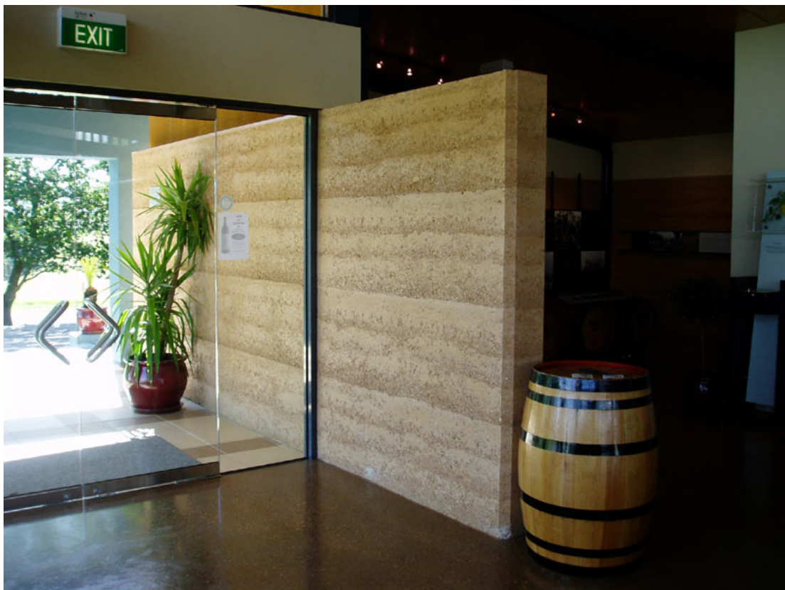
Detail of Rammed Earth wall
