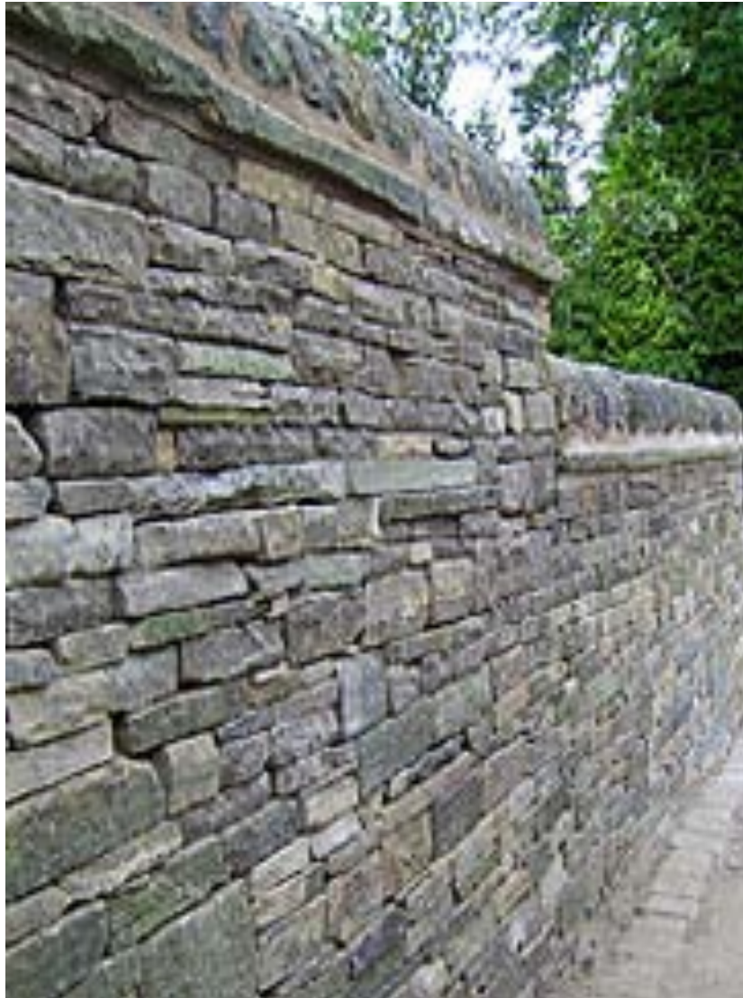
Detail of dry Stone Walling
