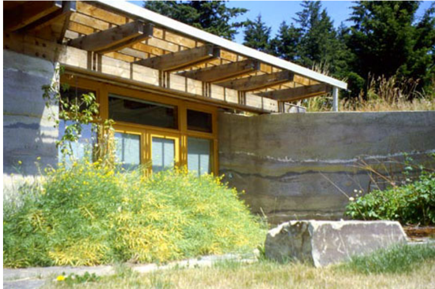
Rammed earth walls extending out into landscape
