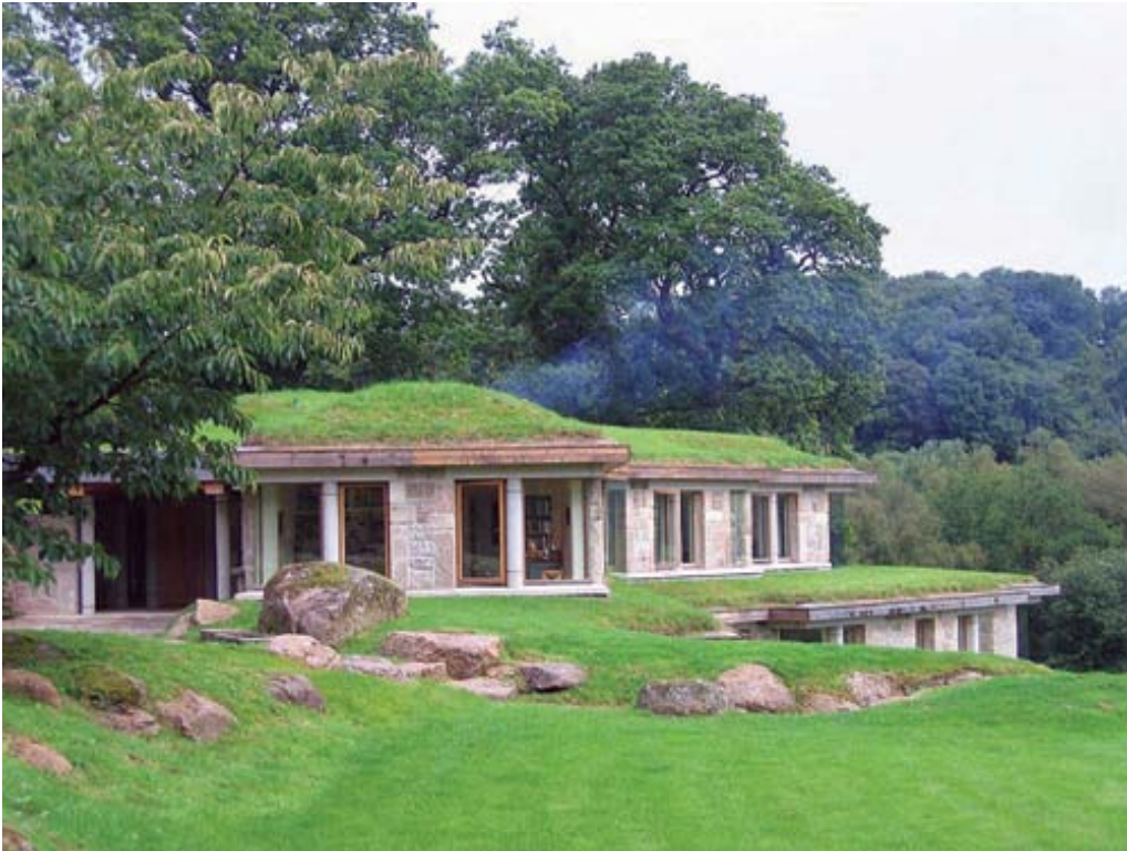
Image of sedum roof
