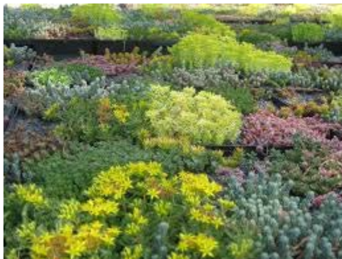
Detail of sedum roof
