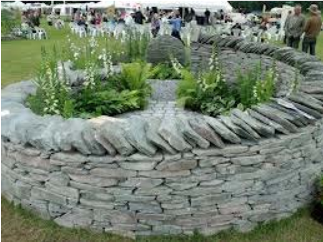
Example of Dry Stone Walling
