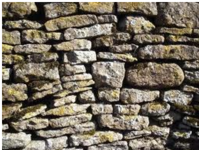
Detail of Dry Stone Walling
