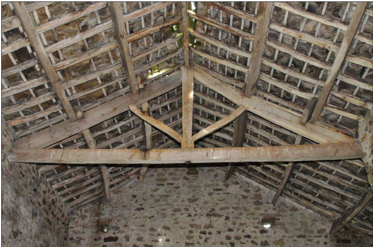
Photo 8: North-west roof truss, with mixture of timber types
