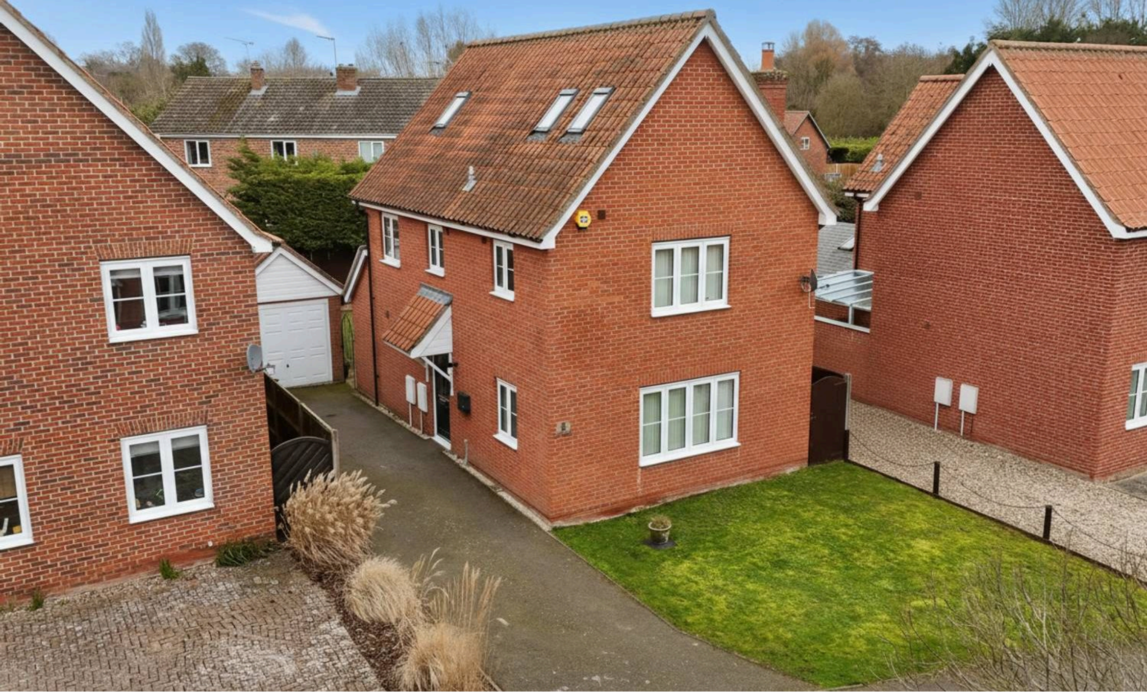
Waterside Gardens, Newton Flotman - NR15 1PA
