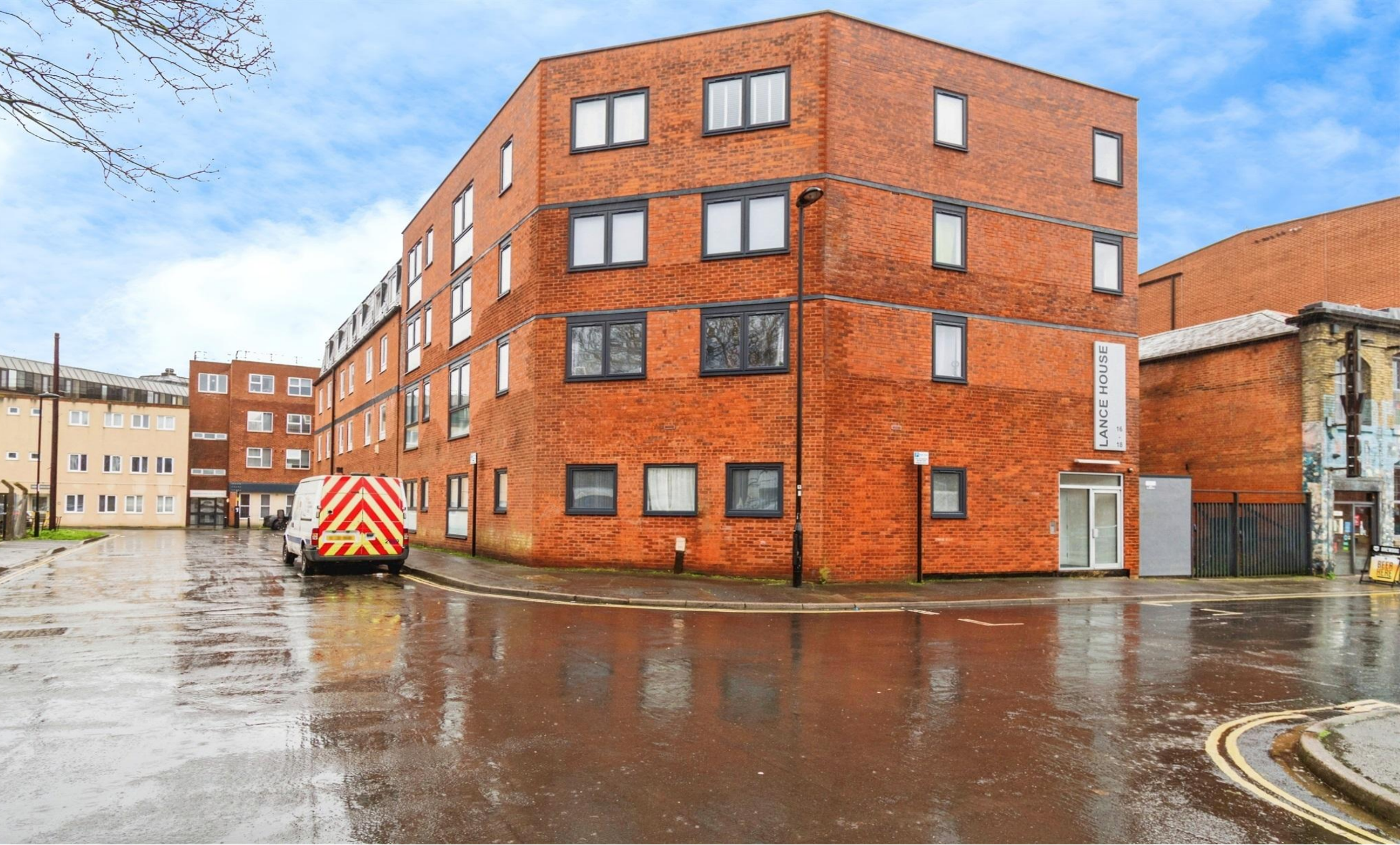
Lance House, Upper Banister Street, Southampton SO15 2EF
