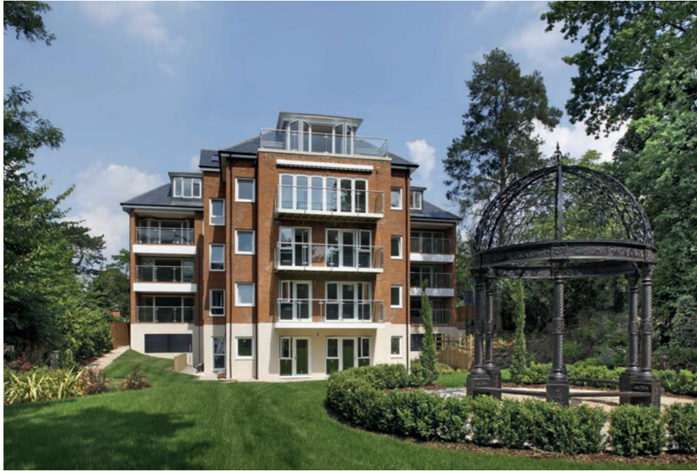
Carisbrooke House, Northwood.
