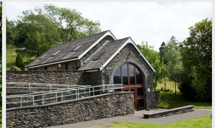
Biomass Fuel Store
