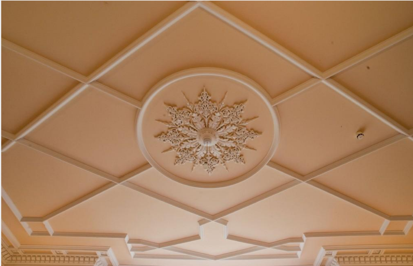
Ceiling in Reception Room/Kitchen
