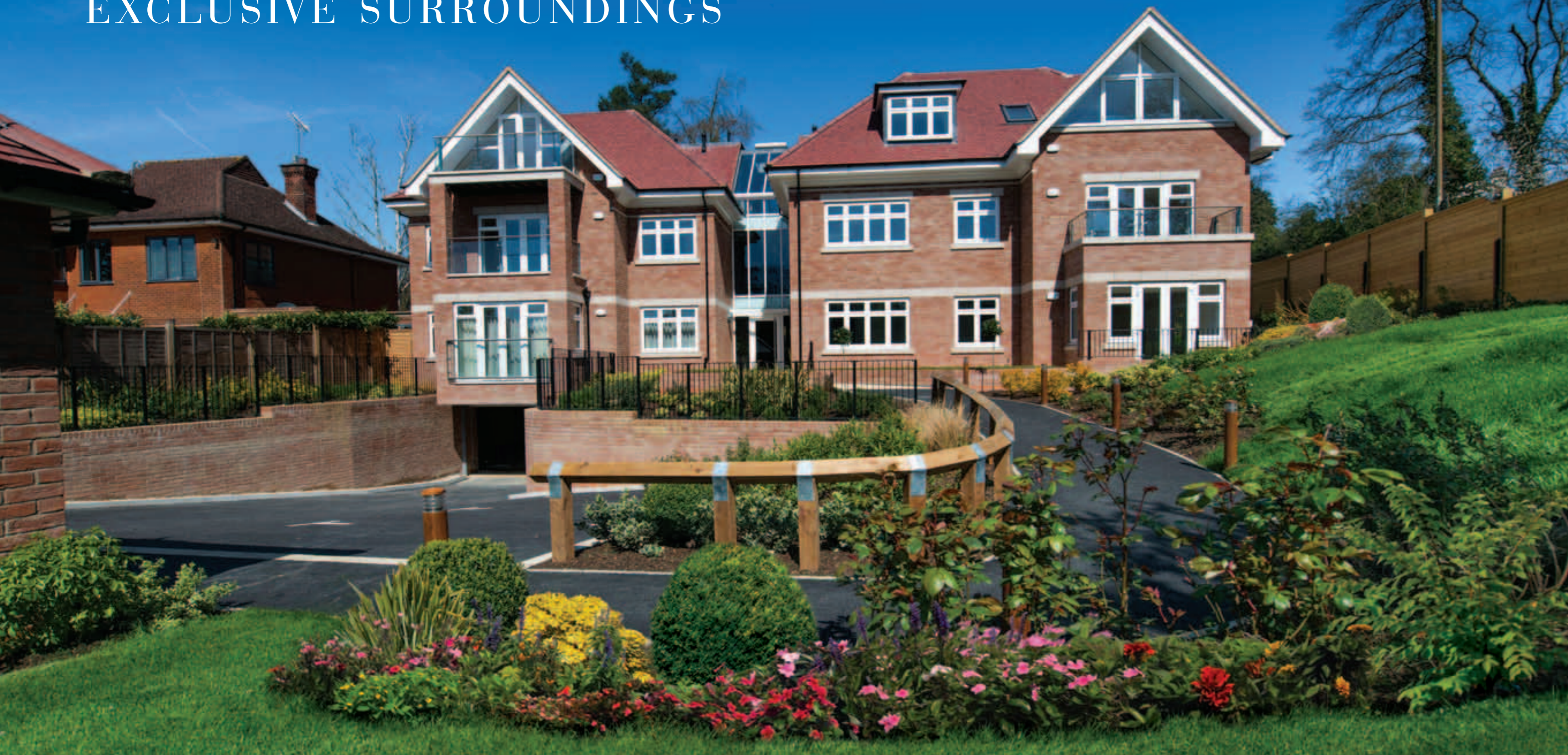
Photograph of Brookmans Manor from the main entrance on George's Wood Road.
