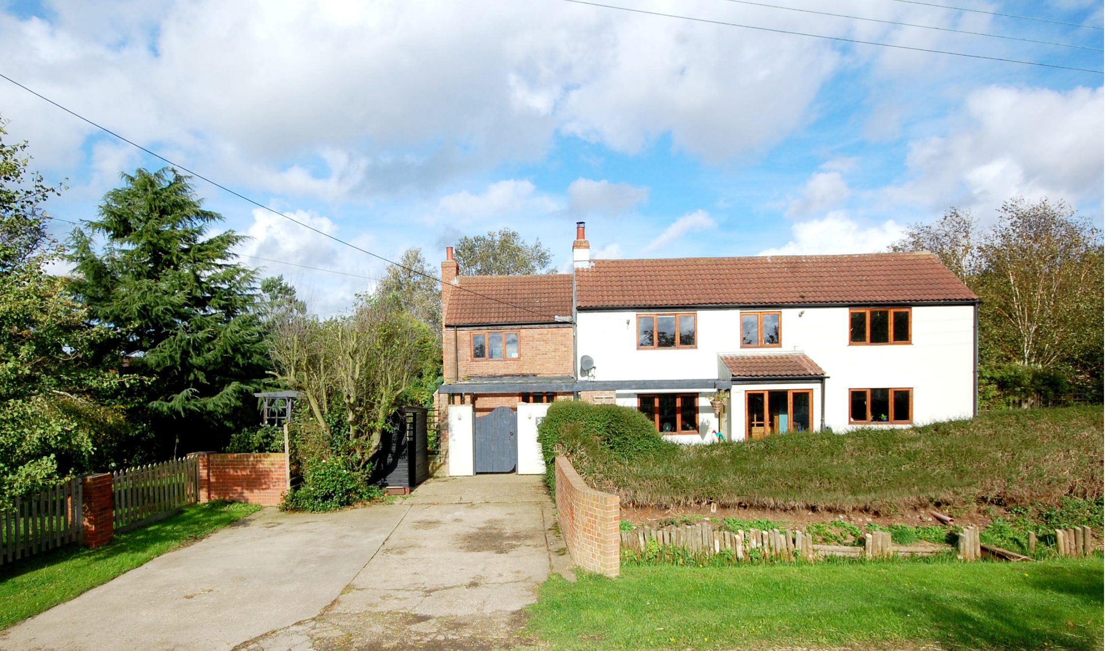
Bridge Cottage Gayton-le-Marsh LN13 0NS
