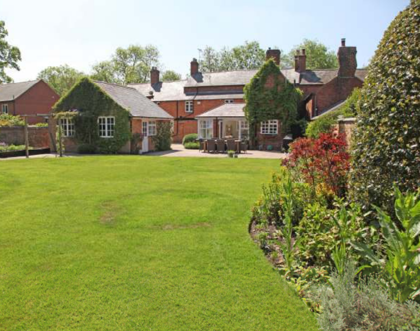
VIEW TO THE FRONT
